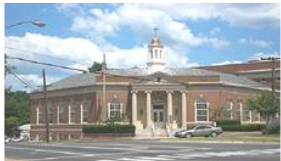
The Robert B. Weiss Center is home to the Town's Human Services Department. The large Colonial and Classical Revival building was originally built in 1931-1932 as the primary U.S. Post Office in Manchester.
